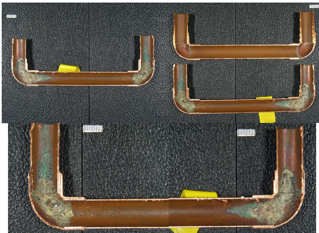
Figure 2: Cross-section views of soldered joints (photo credit: US EPA/ORD)
