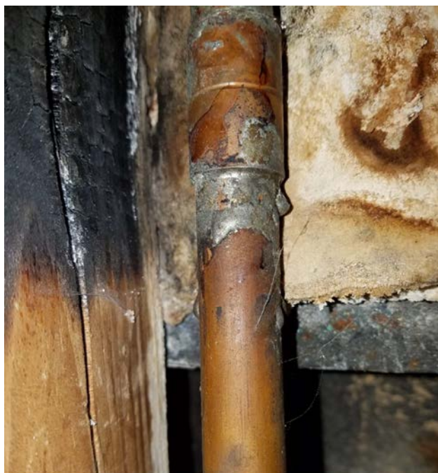
Figure 1: Leaded solder copper joint (photo credit: US EPA/ORD)
