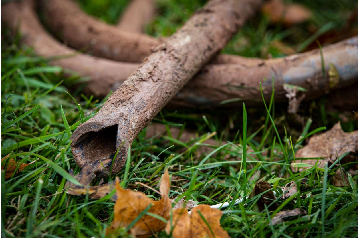
Figure 7: Lead service line (photo credit: US EPA/ORD)
